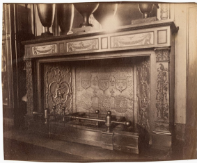
Picture #1 : Eugène ATGET (1857-1927), Egyptian room fireplace mantel with its complete hearth in cast iron, Louvre Museum. The fireback is only the plate in the back.
