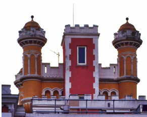
Castellated towers, château des Ollières.
